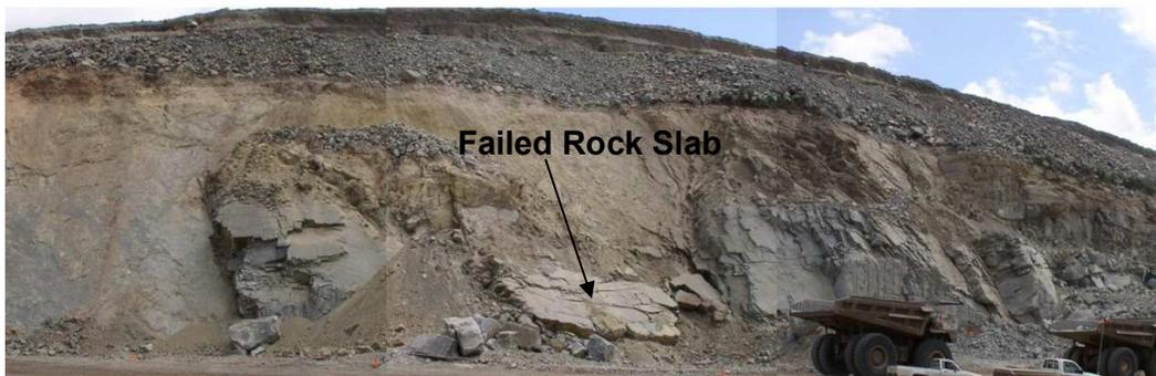
Figure 4: Small Rock Slab Failure
